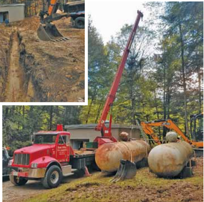
Left: Well # 4 rehab during construction Right: Well # 4 pump removal and inspection
