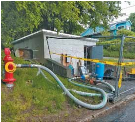
Left: Bypass pumping at Notch Road pump station during pump replacement
