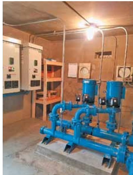
Right: Notch Road pump replacement completed
